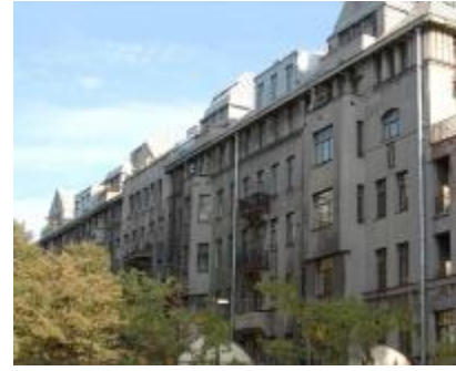
Nekrasova 58-60, residential compound of Basseiny Partnership
