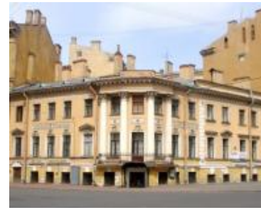
Gagarinskaya 8/4, Apartment house
